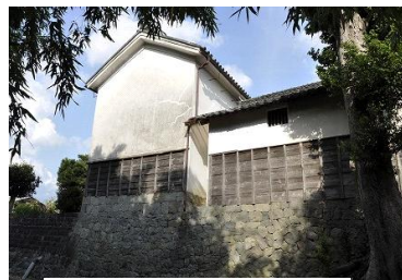
High Stone Wall (Mainakajima, Anabuki Town, Mima City)
